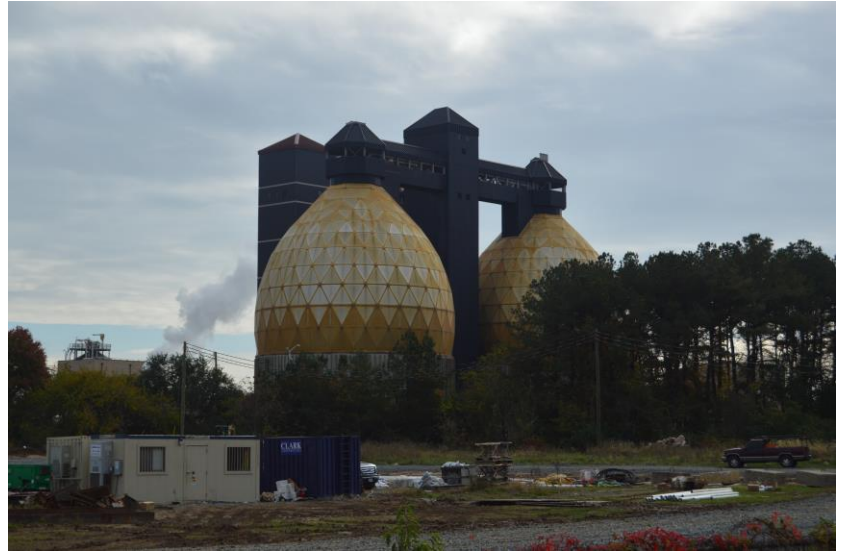
Maryland's largest sewage plant, the Back River wastewater facility, discharged 29 percent more nitrogen water pollution than permitted in 2016. Baltimore officials said in October 2017 they completed a $263 million upgrade to the plant which should be fully tested and online by December 31, 2017.
