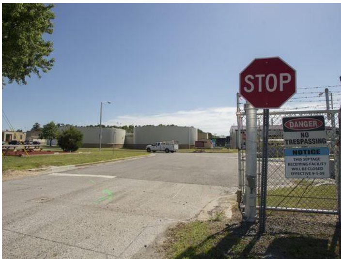
The Salisbury Wastewater Treatment Plant has a long history of water pollution violations, including in 2016 for discharging four times more nitrogen than the permitted limit and in 2017 for releasing at least three times too much. An upgrade to the plant is behind schedule.
